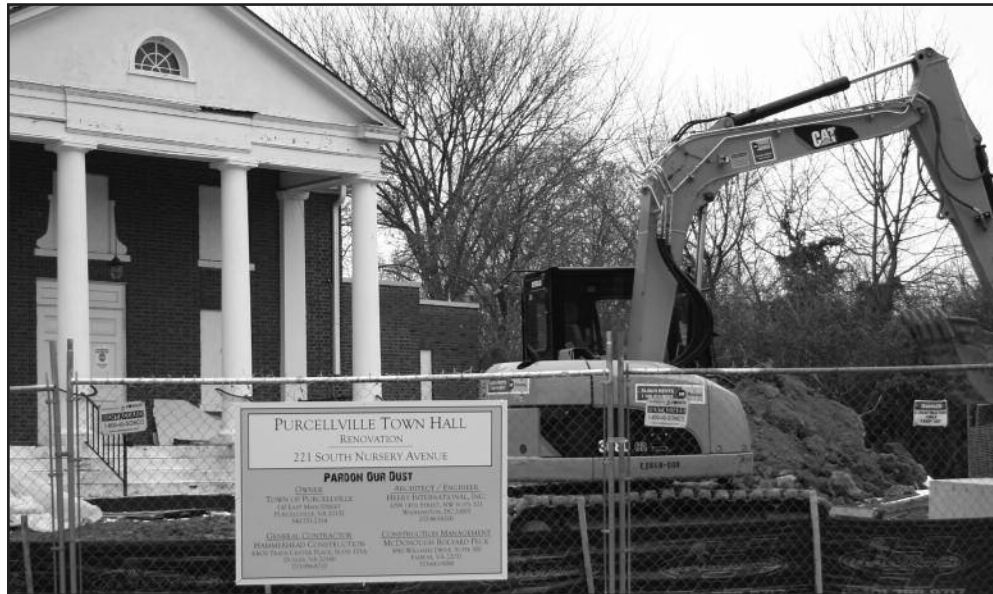
The old Purcellville Baptist Church building under construction.
