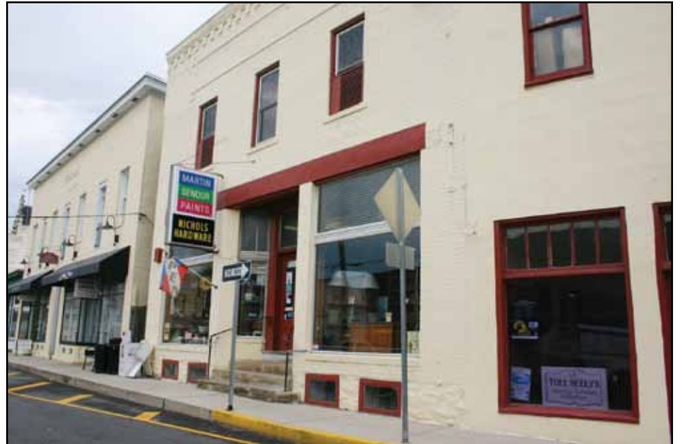
Historic District streetscape, anchored by Nichols hardware.
