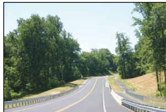
The Town of Purcellville took by Quick Take approximately 7-1/2 acres of Sam Brown's Crooked Run Orchard for the Southern Collector Road. This divided Brown's property in two, leaving neither him nor his customers safe access to his peach orchard (no cross walk and no path for his tractor). The town left approximately the 16-acre adjacent O'Toole property untouched, for future commercial/residential growth.
