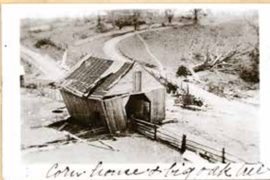
1929 tornado damage to cornerrib and old oaks on the Phillips Farm.
