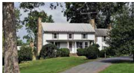
Trough Hill Farm Middleburg, Virginia $2,450,000
