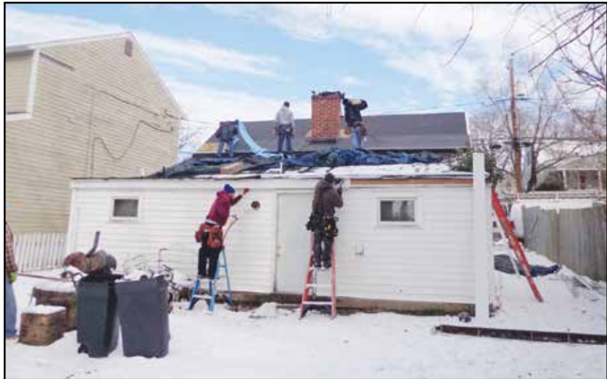
Replacing roof of house from a previous year.
