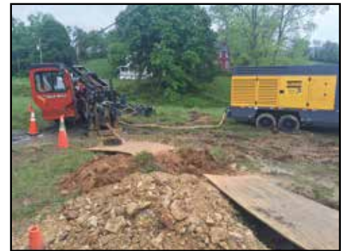
Fiber optics cable work in the yard of Christopher Griggs.
