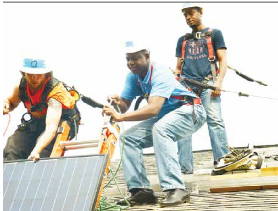
Purcellville Mayor Kwasi Fraser, center, along with volunteers, installs solar panels.
