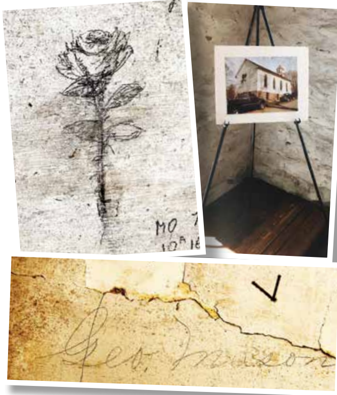
One LPS grant helped stabilize plaster walls in an Oatlands garden shed containing old signatures and sketches. Another grant helped restore original flooring in Waterford's John Wesley Community Church.
