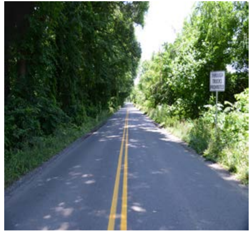
The two-lane Rt. 611/Purcellville Road borders the Warner LLC land on the west side.
