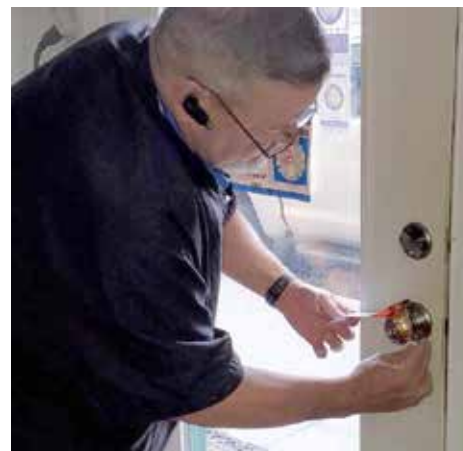
Darrell Furr covers the entrance door knob with copper.
