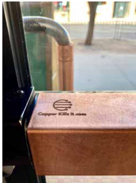
Horizontal and vertical copper covered push/pull bars
