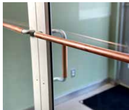
Copper covered push bar and pull bar on a restaurant door
