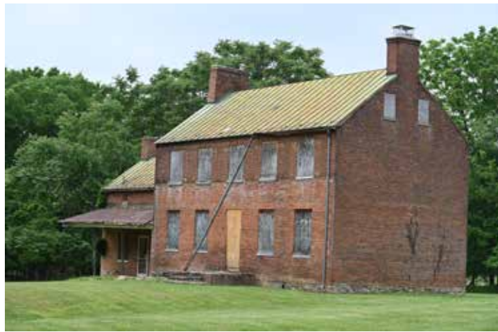
House on Aberdeen property
