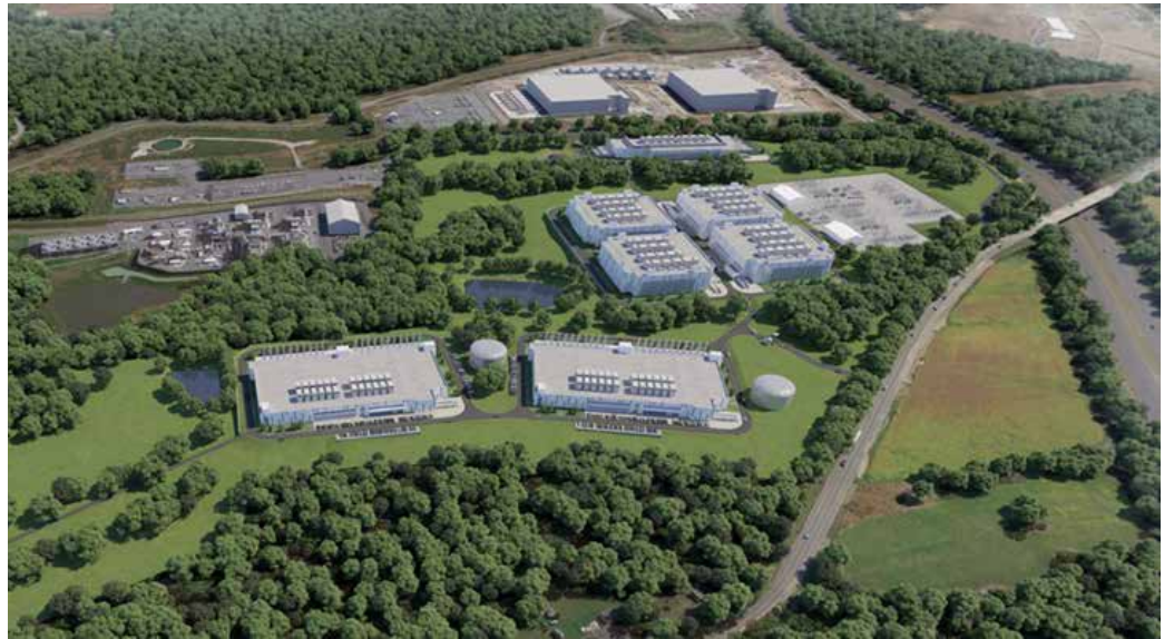
A rendering of TA Realty's data center campus in Leesburg. Courtesy/TA Realty
